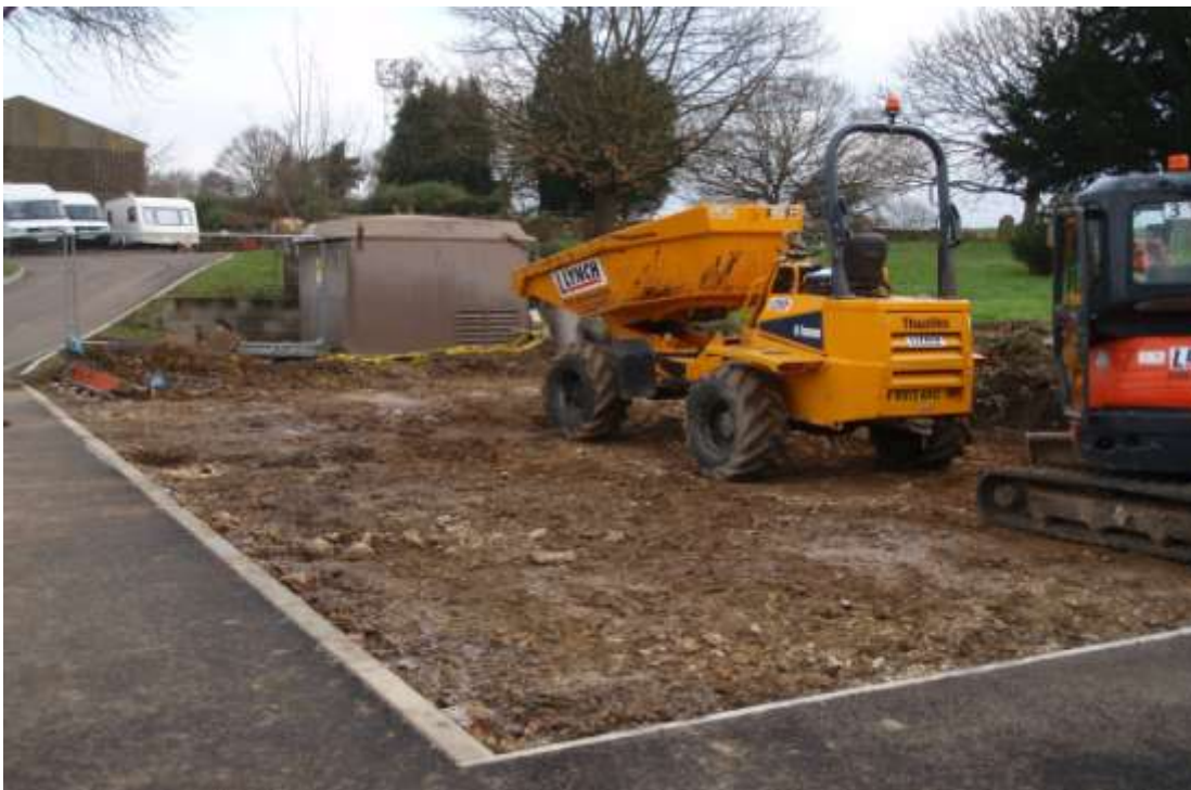
Plate 3. General view of site after removal of barn (looking north)
