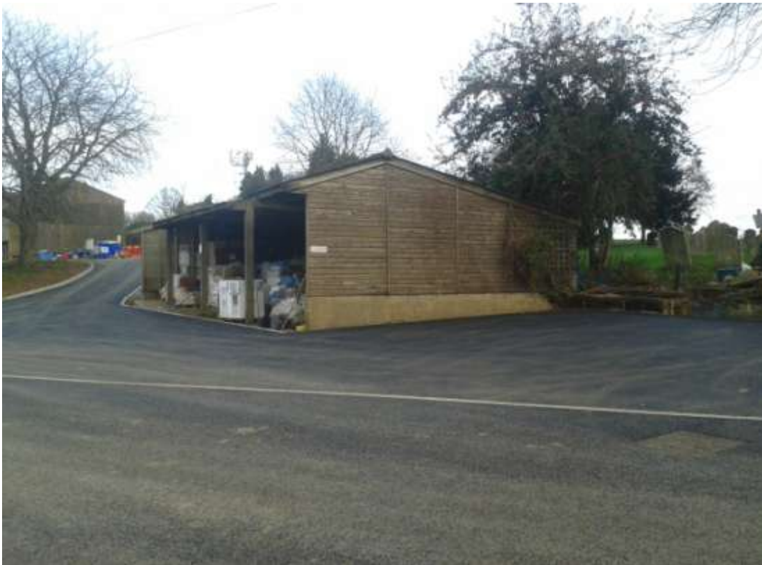
Plate 2. General view of site showing existing barn before demolition (looking north)
