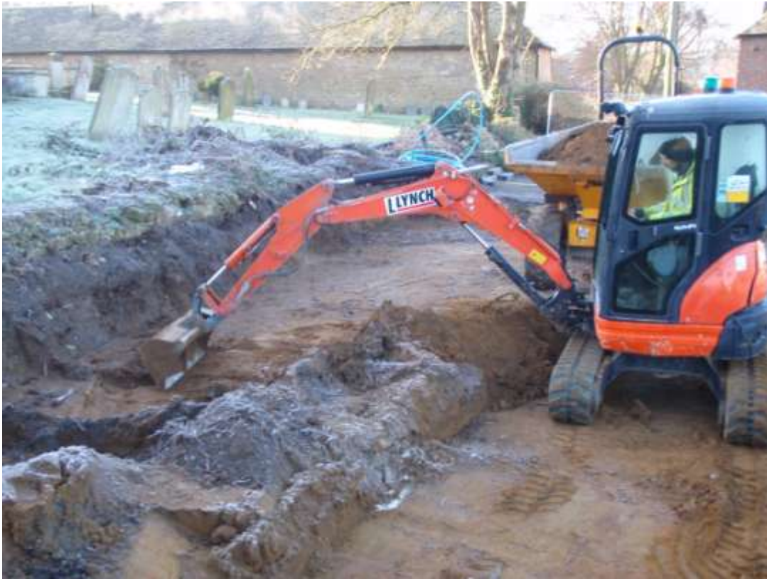
Plate 4. The site showing reduction of site (looking south-east)
